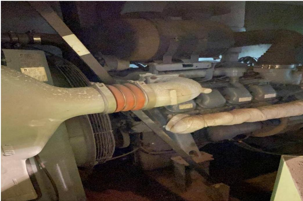
A photograph showing the engine and soundproofing cover for generator #2. Similar to generator #1, a large, light-colored, conical soundproofing cover is positioned on the left side of the engine. The engine is a complex mechanical assembly with various pipes and hoses. The unit is housed within a green-painted metal enclosure.             |    |
