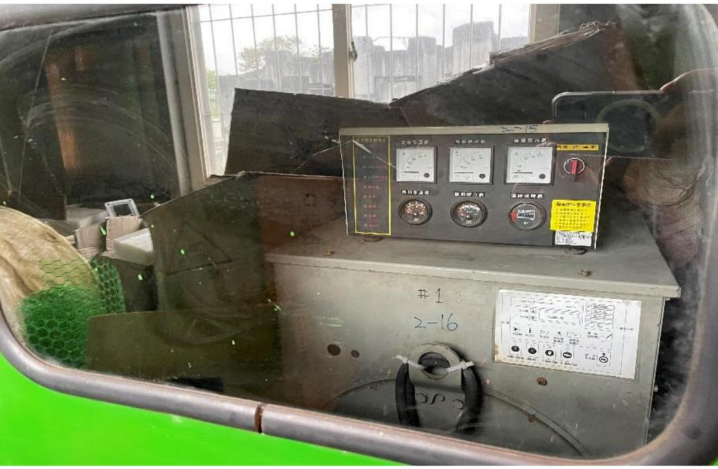
A photograph of the control panel for generator #2. The panel is a grey metal cabinet with a control panel on top. The control panel features several analog gauges, switches, and a red emergency stop button. Below the gauges, there are some handwritten markings: "#1" and "2-16". The panel is situated inside a green-painted metal enclosure. |    |
